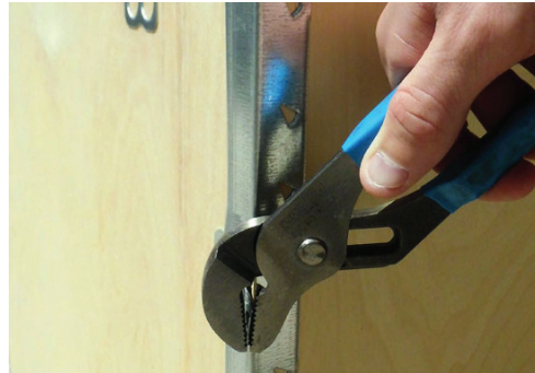
Figure 6: Flattening the tabs with channel locks will allow the wall panel pairs to uncouple more easily and facilitates the eventual reuse of the crate.
